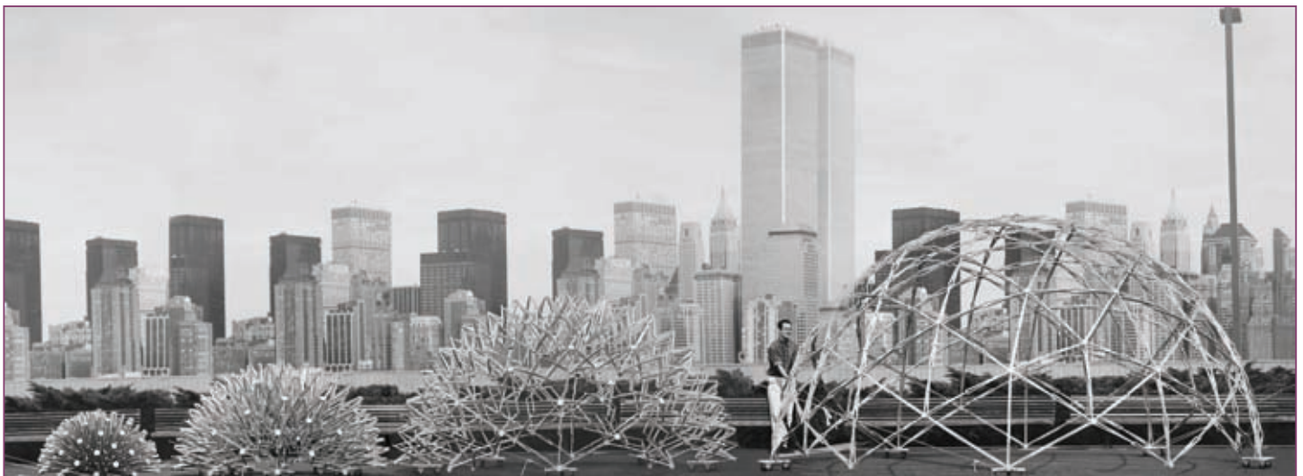
Chuck Hoberman and his transformable geodesic dome showing stages of transformation from 16 inches to 6 foot wide.
