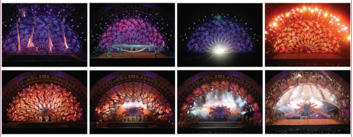
The transformable stage used throughout the 2002 Olympics held at Salt Lake city. Constructed of sand-blasted structural aluminium, fibre-reinforced polycarbonate sheets and more than 13,000 stainless steel connecting pins, the arch retracted in a transforming motion, like the iris of an eye. It stands 36 feet high and 72 feet wide, with 96 structural panels, each 9 feet by 5 feet, and more than 4,000 individually machined pieces. The arch was operated by two 30-horsepower motors controlling eight separate cables.
