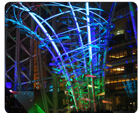
These metal atrium trees were designed in Cobalt and fabricated in China, using Cobalt as a "production language" easily understood by non-English craftsmen.
