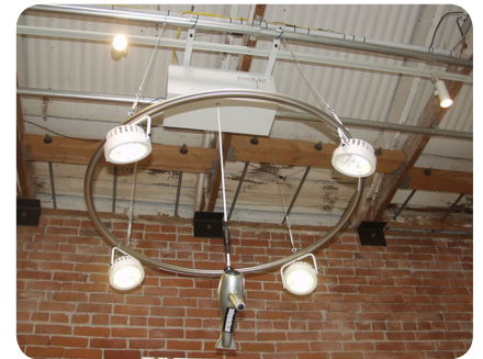
Above and below: the SpectraLights high-lumen, low energy lighting system.
